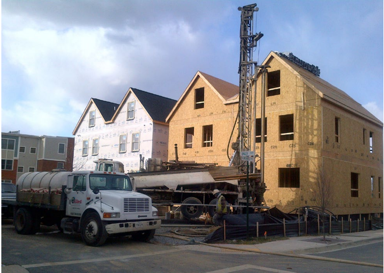
Geothermal well installation & SIPs envelope construction NEXUS ENERGY HOMES
